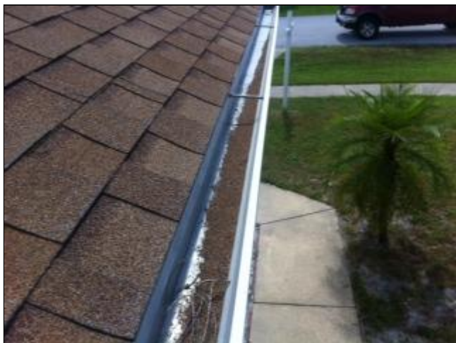
1.3 Picture 1 roof drainage
