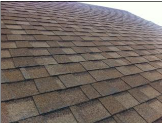
1.0 Picture 3 roof covering
