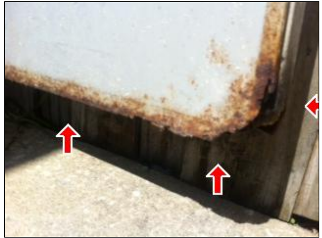
2.1 Picture 2 base of service door
