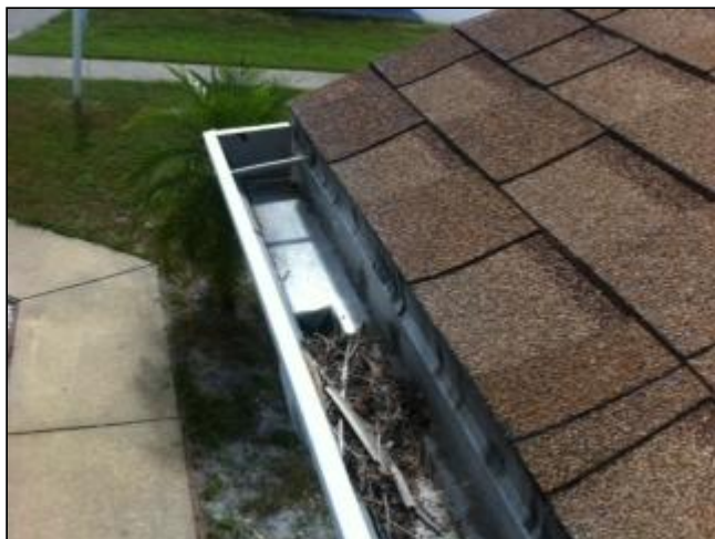
1.3 Picture 2 roof drainage
