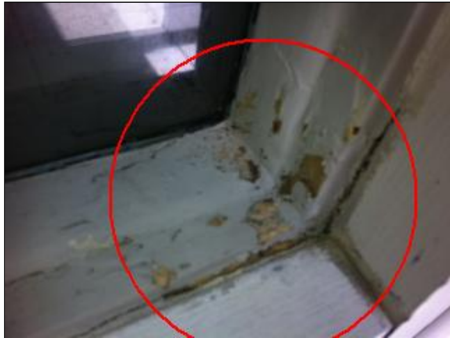
2.2 Picture 1 fixed light at entry door
