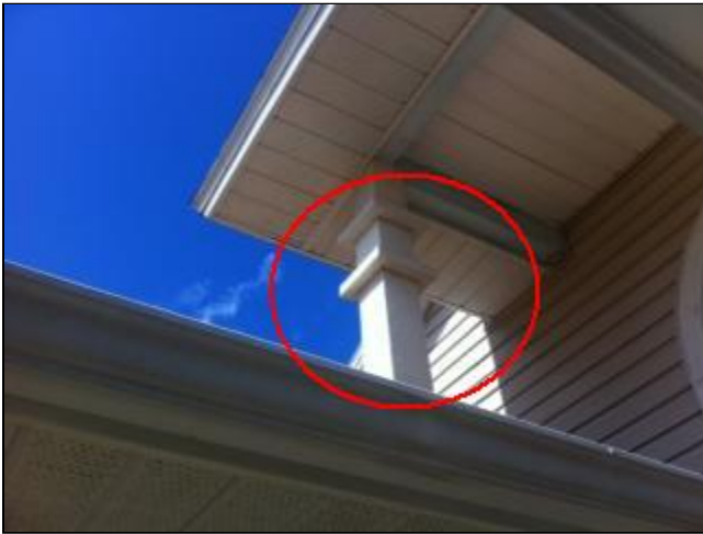
5.2 Picture 1 portico support beam
