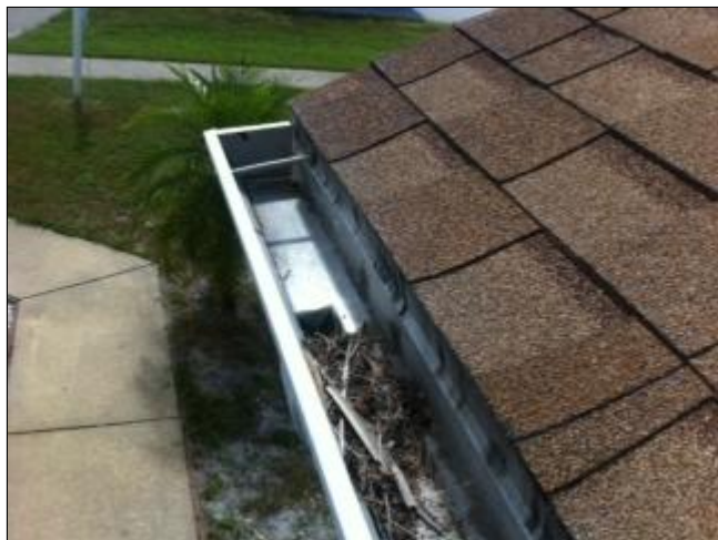
1.3 Picture 2 roof drainage
