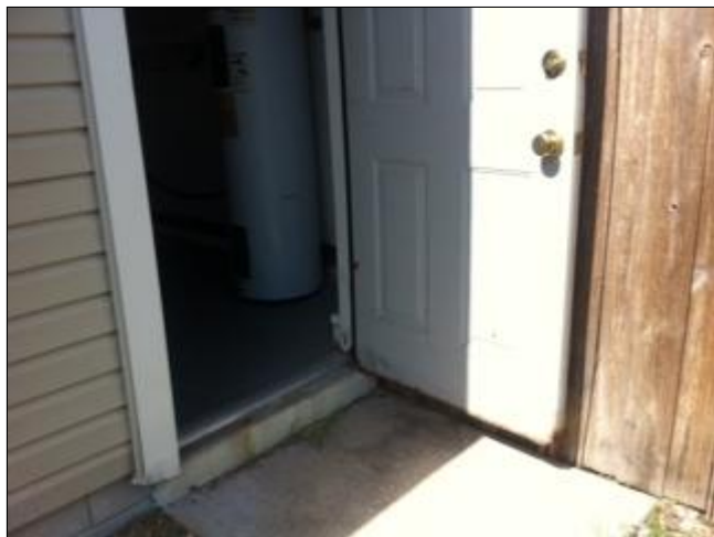
2.1 Picture 1 exterior service door to garage
