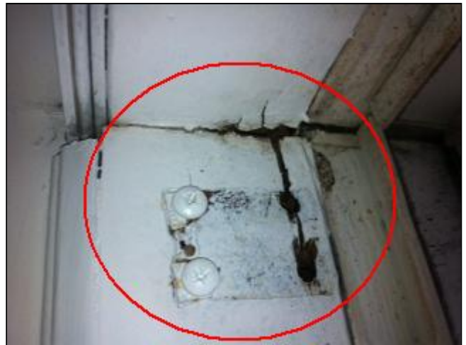
2.1 Picture 4 Front entry door jamb
