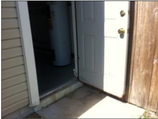
2.1 Picture 1 exterior service door to garage
