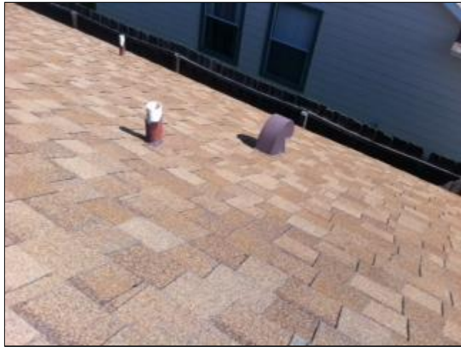
1.0 Picture 2 roof covering
