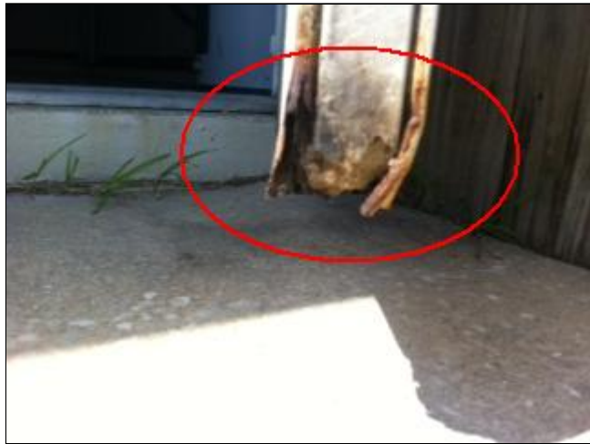
2.1 Picture 3 base of service door
