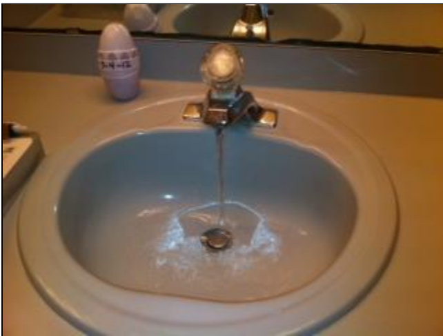
6.1 Picture 1 hot water distribution
