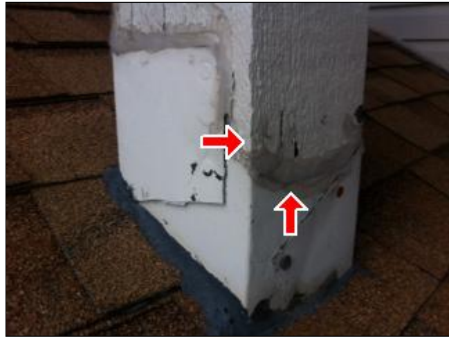
5.2 Picture 2 portico support beam
