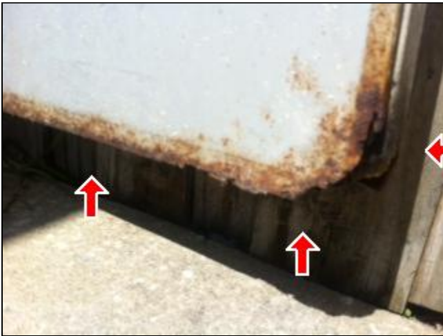
2.1 Picture 2 base of service door
