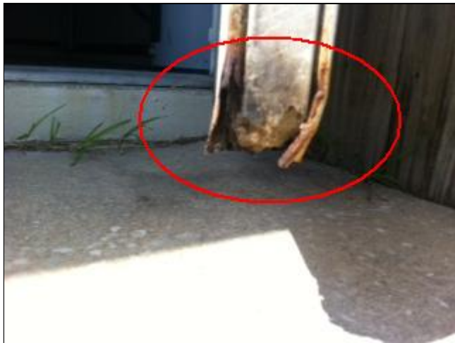
2.1 Picture 3 base of service door
