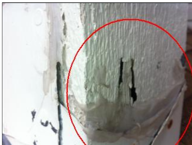
5.2 Picture 3 portico support beam
