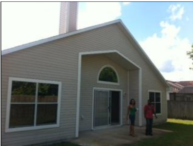
2.0 Picture 3 rear elevation
