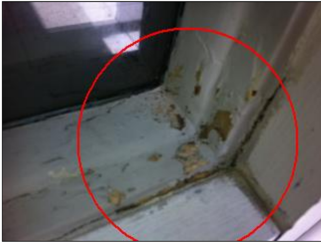
2.2 Picture 1 fixed light at entry door
