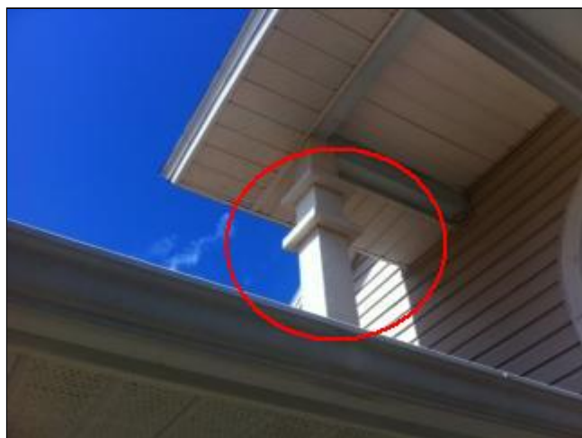
5.2 Picture 1 portico support beam
