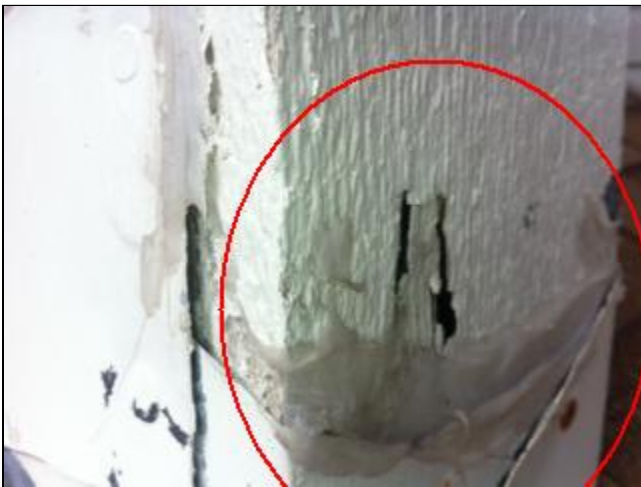
5.2 Picture 3 portico support beam
