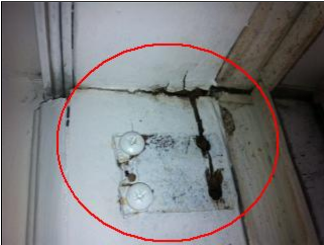
2.1 Picture 4 Front entry door jamb
