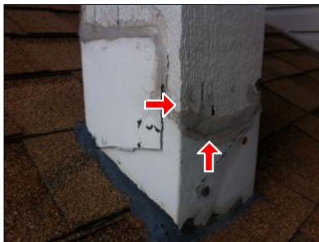
5.2 Picture 2 portico support beam
