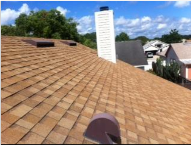
1.0 Picture 1 roof covering
