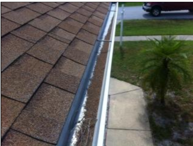
1.3 Picture 1 roof drainage
